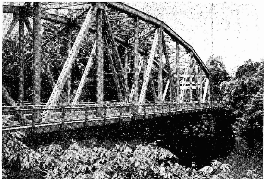
PHOTO #16: Steel bridge above the dam
